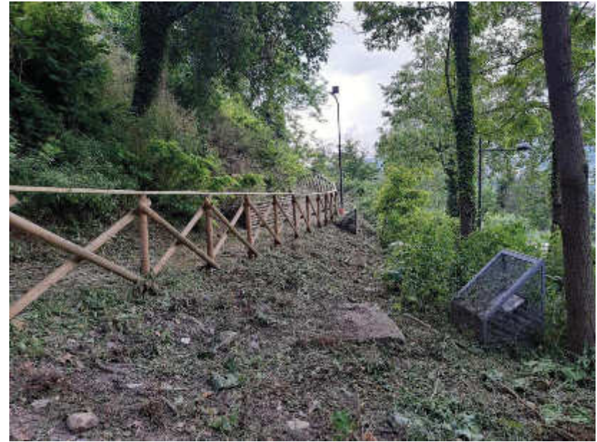
Foto 2.7 – Vista post operam
