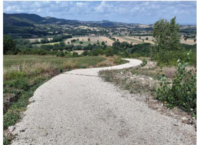
Foto 3.8 – Vista post operam
