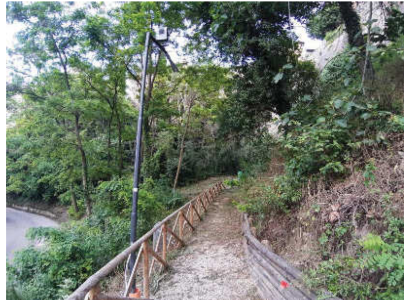
Foto 2.8 – Vista post operam
