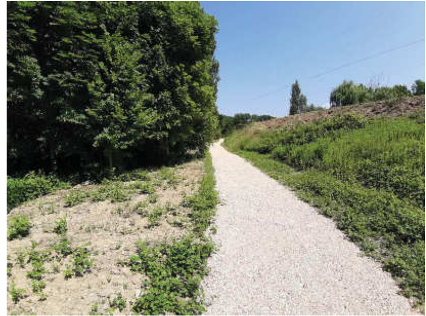
Foto 7.2.7 – Vista post operam
