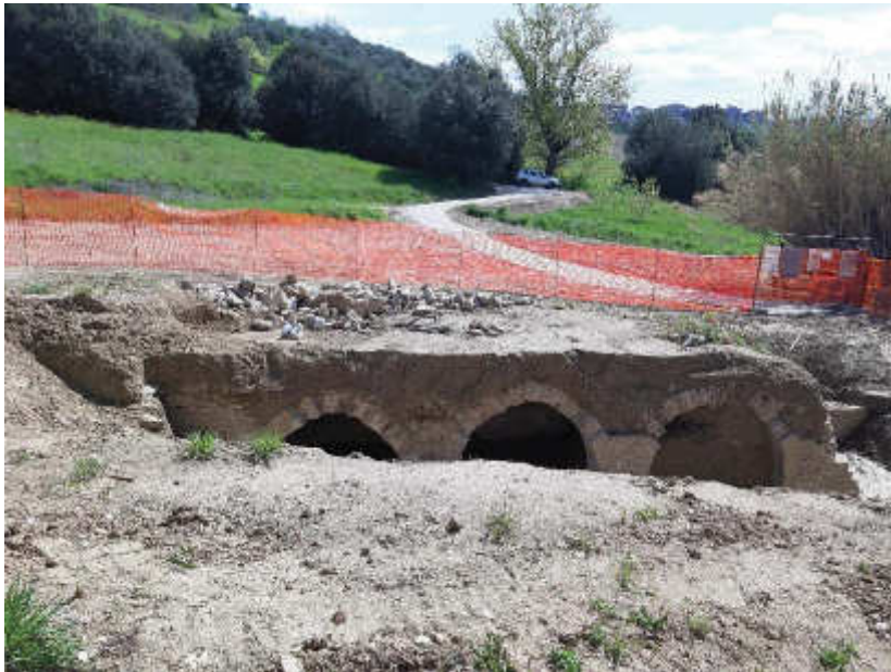
Foto 6.6 – Vista post operam
