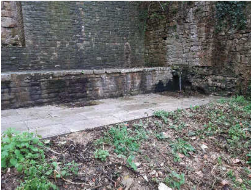
Foto 2.5 – Vista post operam
