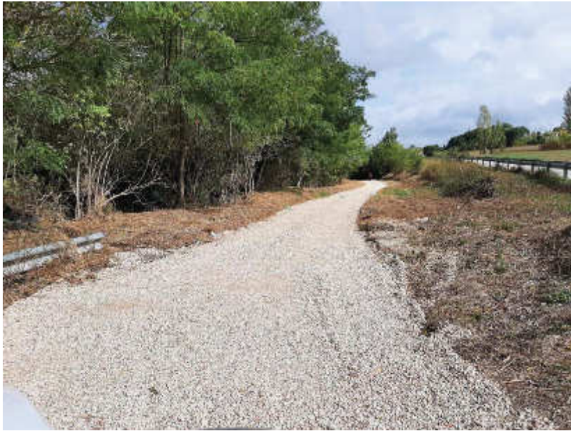
Foto 3.9 – Vista post operam
